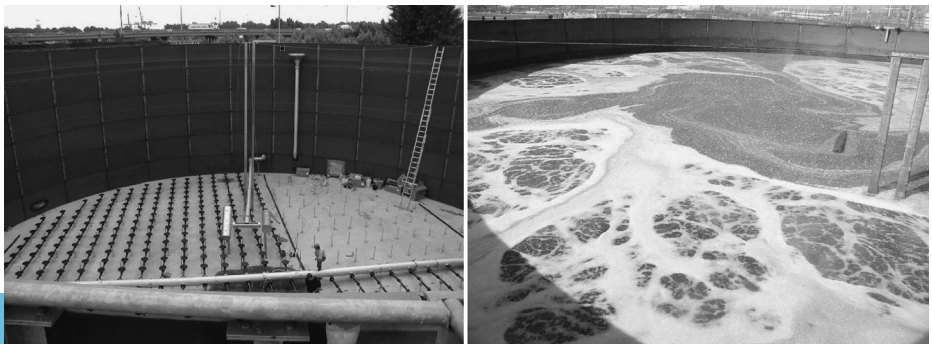
Figure 1 SAT installation under construction (left) and in operation
